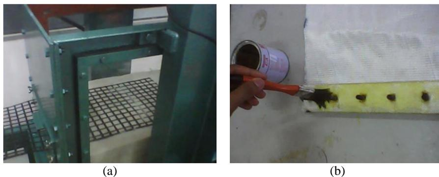
Fig. 2 - (a) installation of geogrid; (b) gluing of the geotextile
