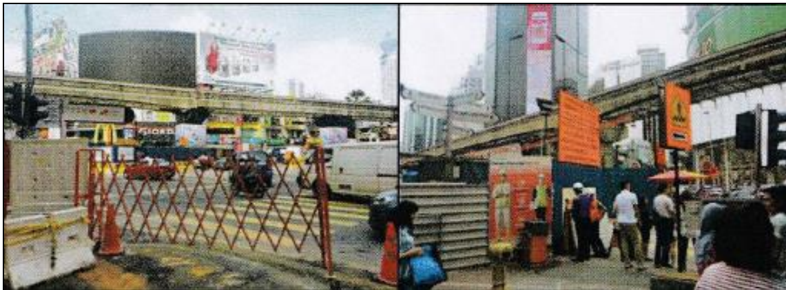
Fig 4 - Surrounding of Bukit Bintang MRT construction site [17]
