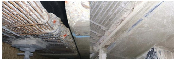
Fig. 3 - Before and after photos of Dean's Brook Viaduct repair work
