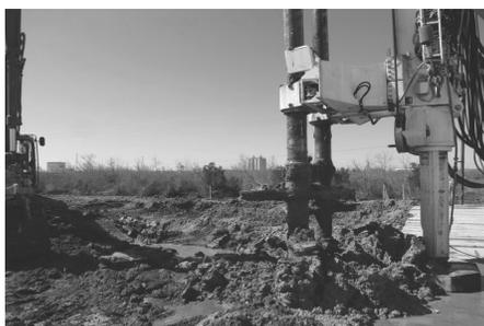
Fig. 20 Deep soil mixing injects cement grout columns deep into poor soil. <http://www.defensemmedianetwork.com>
