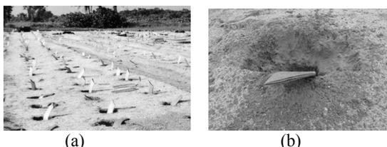
Fig. 19 a) Prefabricate vertical drain at site b) close view of vertical drain.
