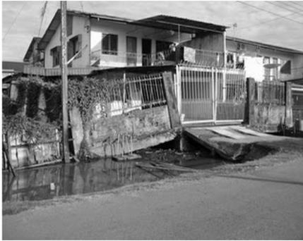
Fig. 16 House settled after a year completion of the construction
