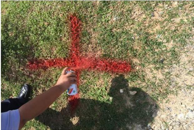
**Fig. 4 - Temporary ground control point that should be in (1m x 1m) size at the Rimba Mas landfill.**
