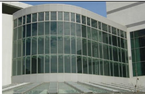
Fig. 4 - Two-storey black wall with vertical glass glazing [11].
