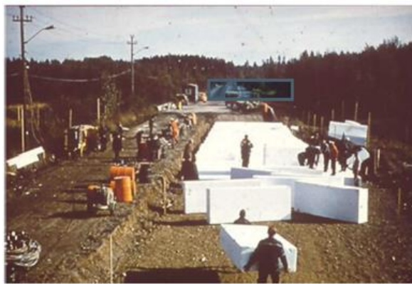
Fig. 1 – Expanded polystyrene (EPS) as a filling material in road construction [7]
