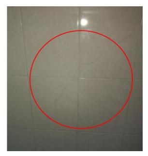
Fig 12 Cracking on the wall finishing
