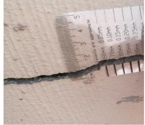
(b) 7mm crack on the wall
