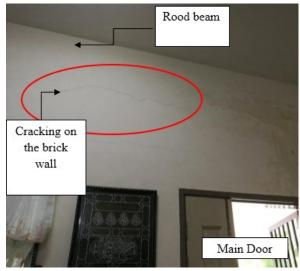
Fig 11 Cracking on brick wall
