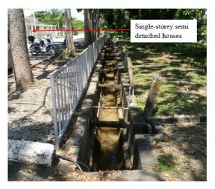
Fig. 3 Concrete drain in front of the semi-detached single storey houses
