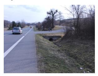
Fig. 5 Rigid culvert headwall (1<sup>st</sup> class road I/52, km 34 - 35).
