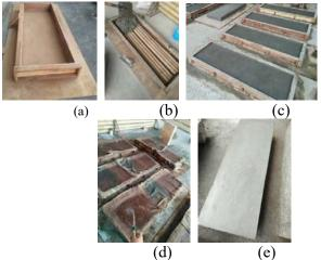
Fig. 3 Bamboocrete Multi-purpose Panel Casting. (a)Wooden formwork (b) Pieces of wrapped bamboo placed in formwork (c) Bamboo casted in lightweight concrete (d) Curing for 28 days (e) Sample Panel
