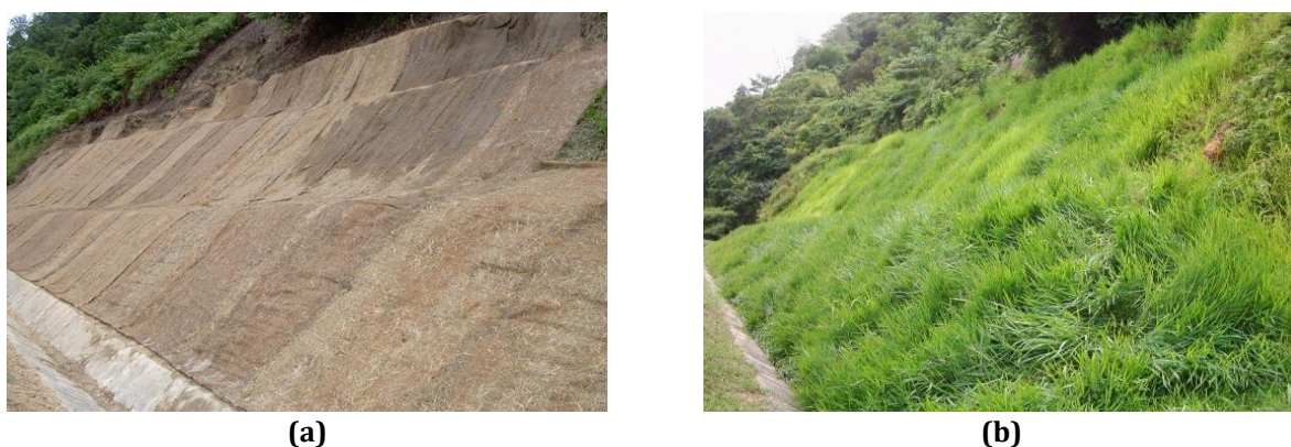
Fig. 4 Vegetation slope (a) Erosion control blanket; and (b) Vegetation of signal grass on slope [20]
