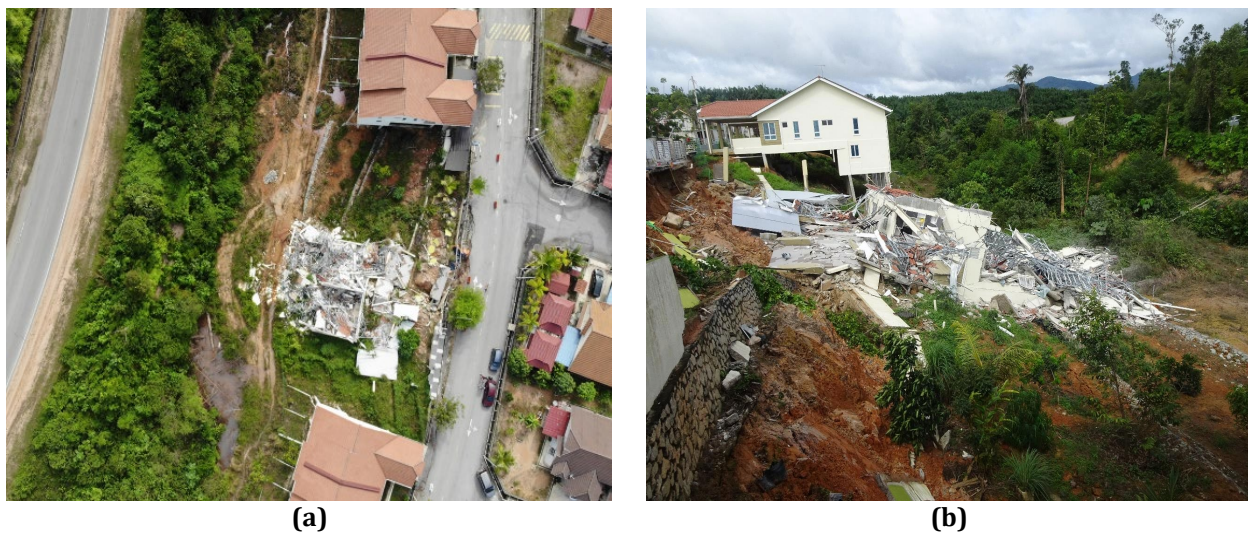
Fig. 1 Landslide area (a) Aerial photogrammetry of the failure area; (b) Collapsed house affected
