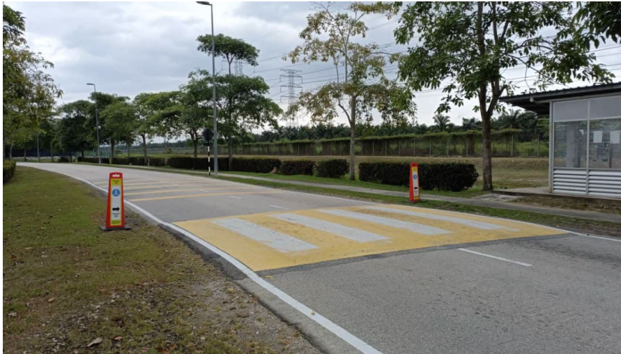
Fig. 1 Raised crosswalk in UTHM campus installed on one one-way street with two lanes
