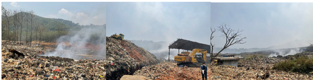
Fig. 2 Condition of Sarimukti landfill fire
