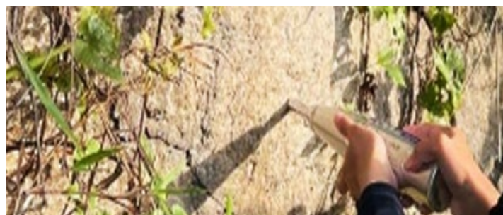
Fig. 3 Collecting rebound data using the Schmidt hammer
