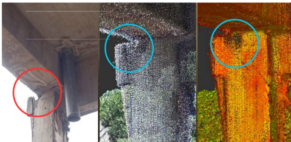
Fig. 10 Comparison of damage visualization on field object and 3D model
