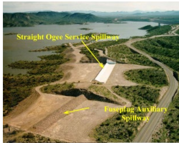
Fig. 2 An emergency spillway with fuse plug (bottom) and an auxiliary ogee spillway (top) at New Waddell Dam [12]
