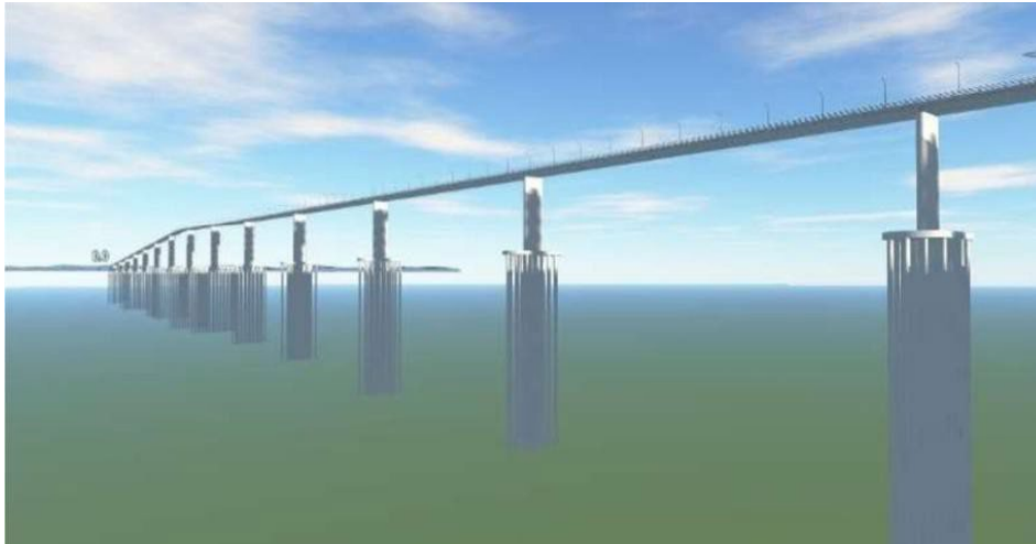
Fig. 7 Muara Lassa Bridge
