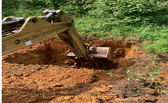
Fig. 2 Excavation work (trial pit) at study area
