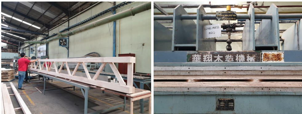
Fig. 1 Fabrication of Sengon OWTJ
