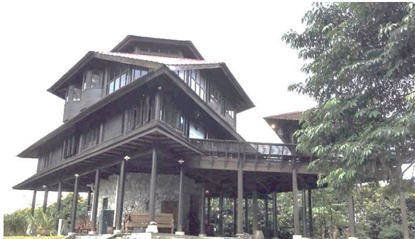
Fig. 9 - Salinger House, designed by architect Jimmy Lim [14]
