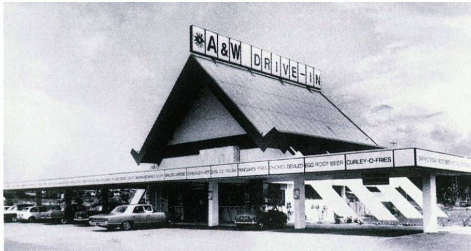
Fig. 6 - A&W Drive-In (1967), the first drive-in in Malaysia, designed by architect Chen Voon Fee
