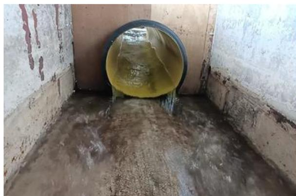
**Fig. 5 - The perforated subsurface drain with smooth inner wall**
