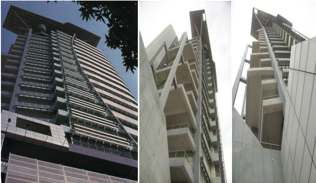
Figure 2: United Malay National Organisation Building (UMNO Tower)
