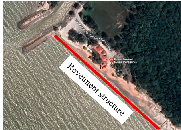
Fig. 2 Natural and hard-engineered defences coexist at Pantai Punggur, Johor
