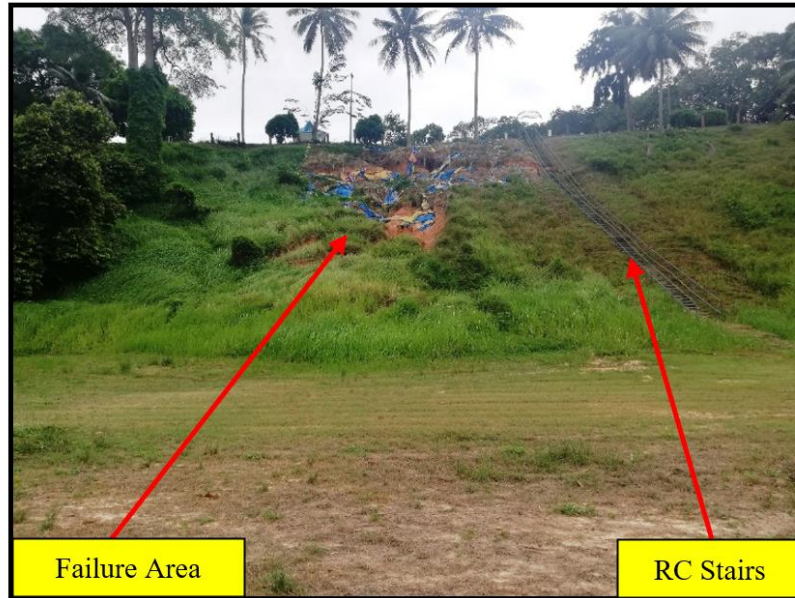
Fig. 4 - View of the slope
