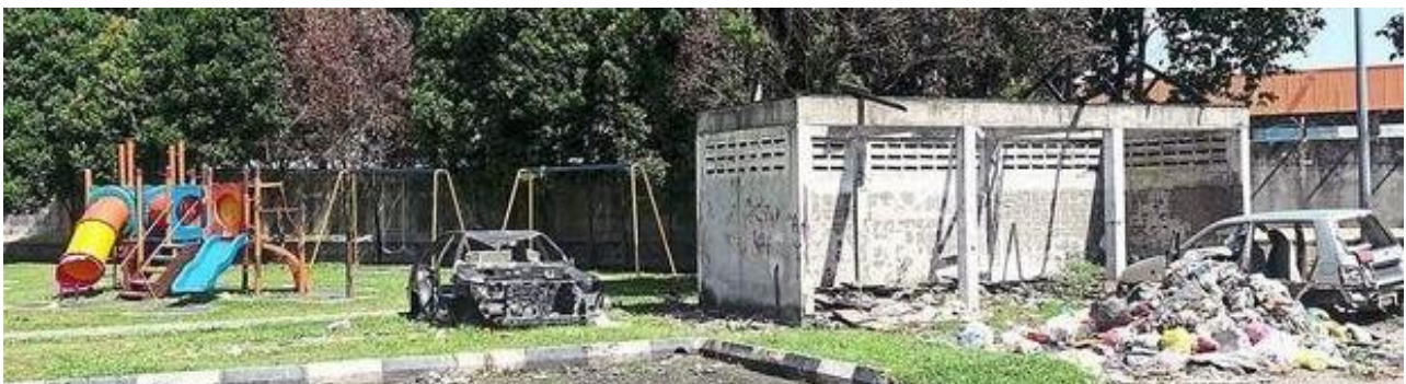
Fig. 5 - Poor and unsafe condition of public area in Public Low Cost Housing Shah Alam (Source: Menon & Zulzaha, 2015)
