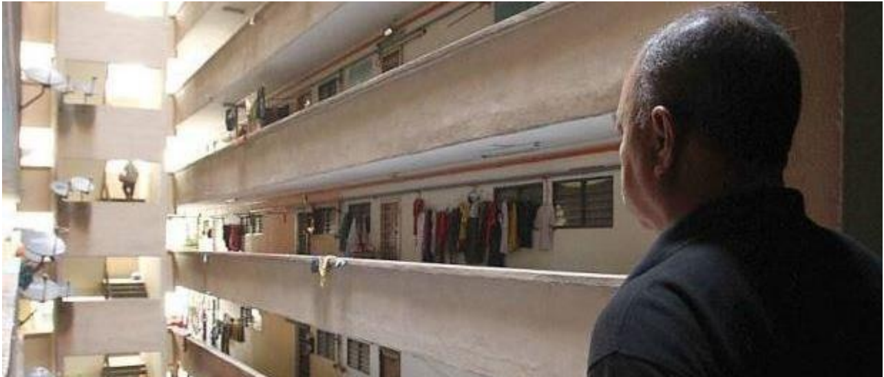
Fig. 4 - Exterior compound in the studied low cost complex in Klang Valley (Source: Menon & Zulzaha, 2015)
