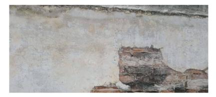
Fig. 8 - Delamination occur after side by side with spalling
