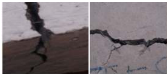
Figure 13: Bridging action of steel fiber on concrete panel
