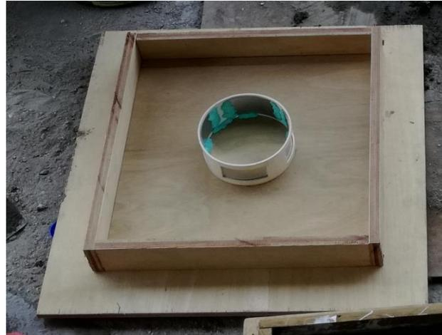
**Fig. 1 - Formwork with pipe sleeve**
