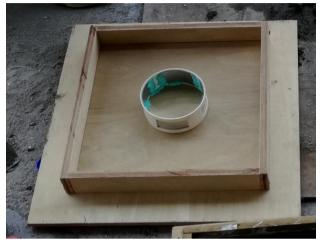
Fig. 1 - Formwork with pipe sleeve
