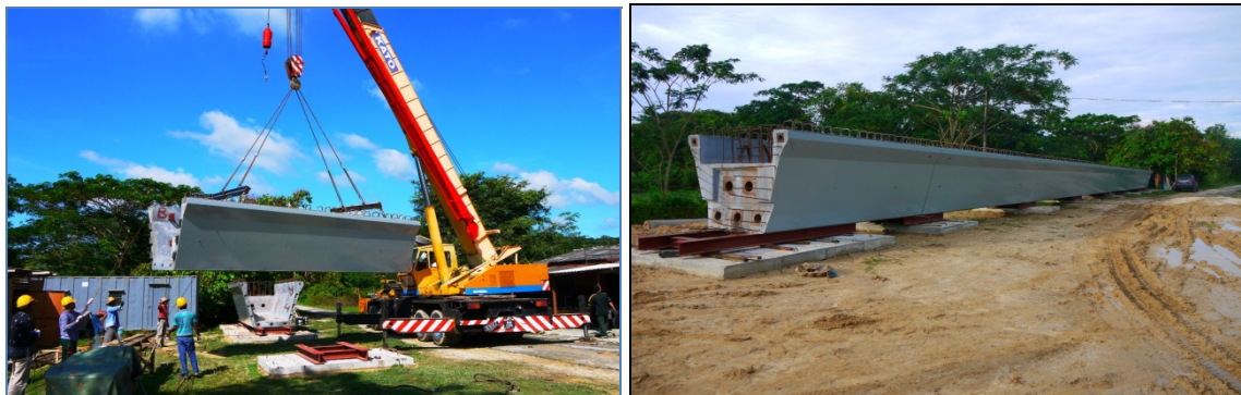
Figure 6: One unit 45 tonnes mobile crane used to assembled the U-segment and (b) full U-girder assembled on site.
