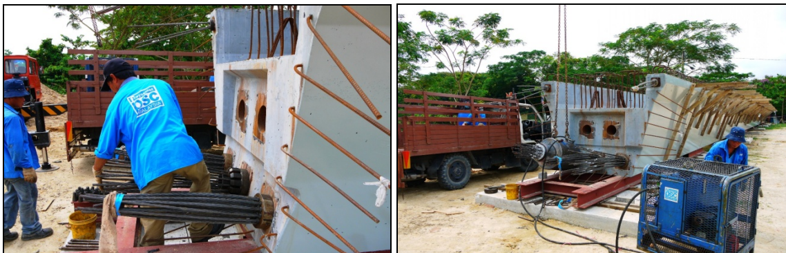
Figure 7: Stressing technician preparing for first stage post-tensioning.
