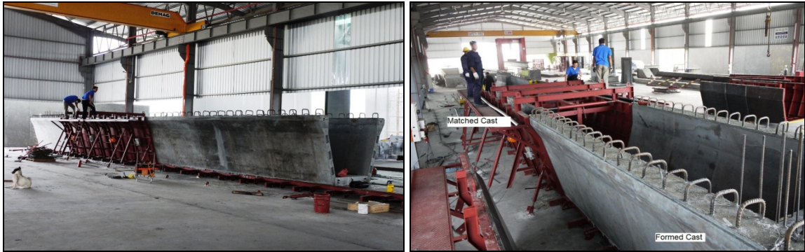
Figure 5: (a) Matched casting of internal segment (b) close up view.
