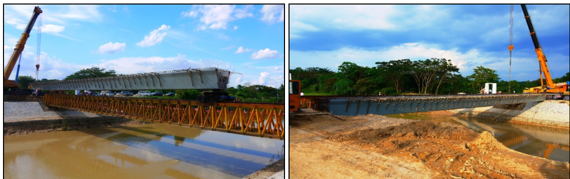
Figure 8: (a) Launching of U-girder using steel A-frame transfer girder, (b) U-girder securely seated on abutments.
