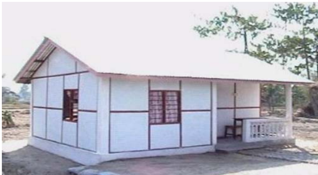
Fig.2.1: 280 Sq.ft house, Stone foundation, Bamboo wall plastered with cement (source:www.habitat.org/ap) [13]
