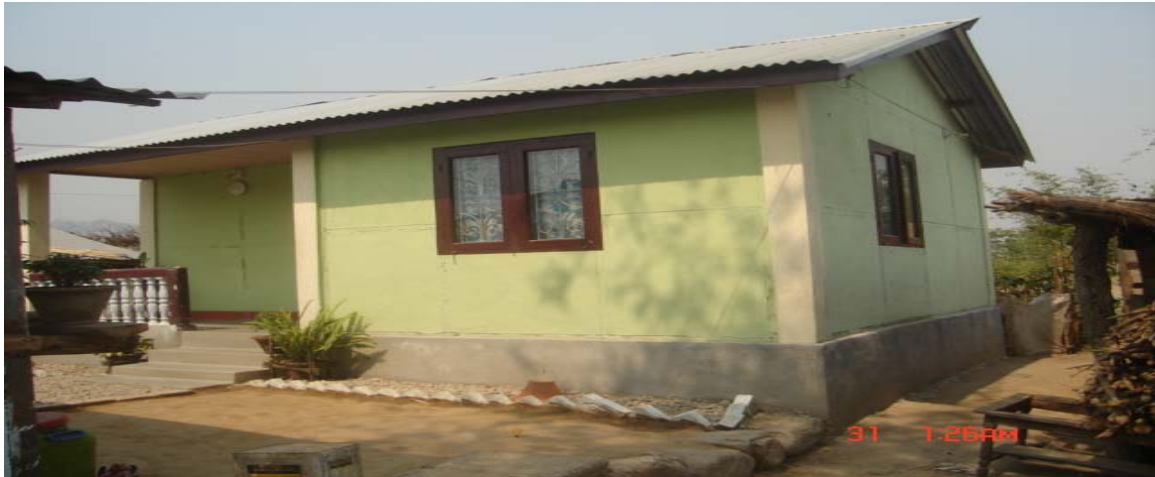
Fig.2.2: 280 Sq.ft. house, stone foundation, Bamboo wall in timber frame (source:www.habitat.org/ap) [13]
