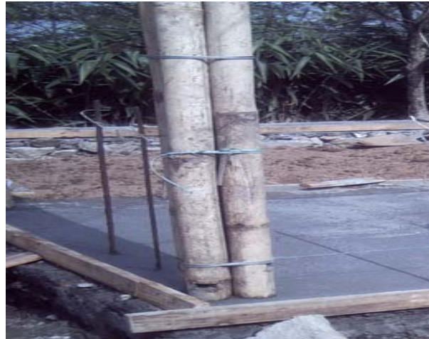
Fig 2.3: Bamboo Column (source:www.habitat.org/ap) [13]
