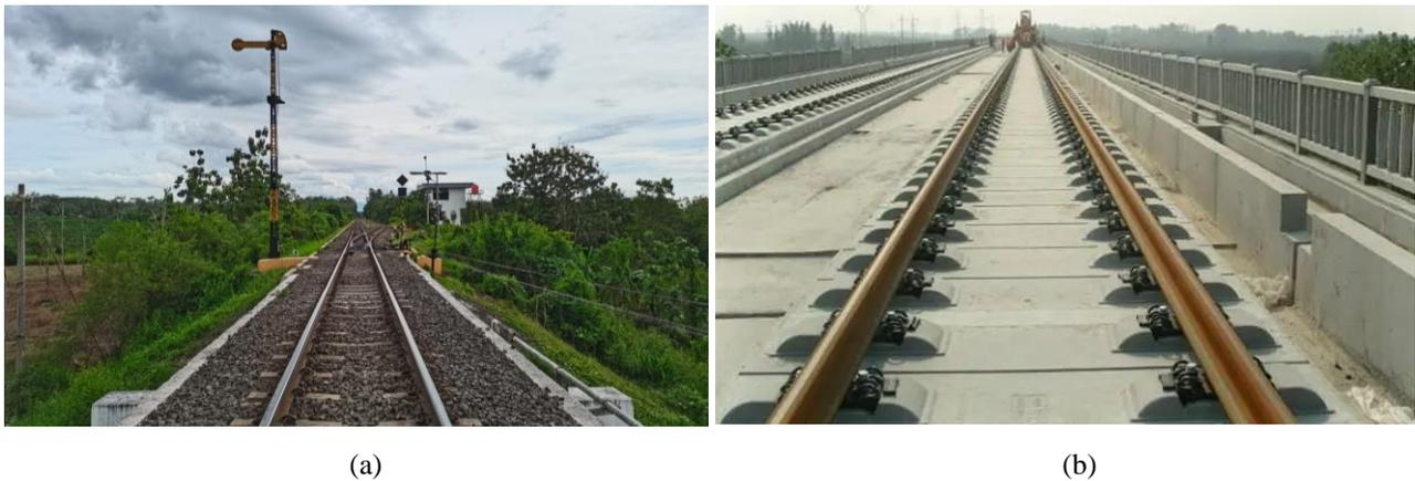
**Fig. 2 - Different types of railway track structure: (a) Ballasted track; (b) Ballastless track**
