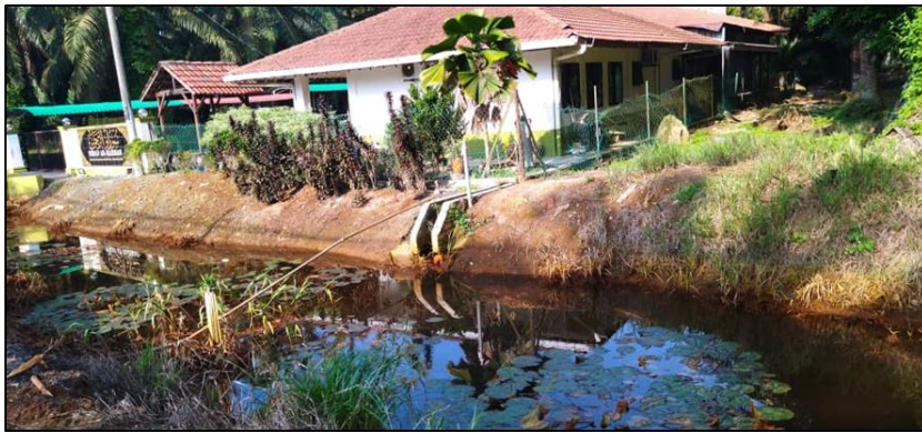
Fig. 3 - Industrial area (S2)
