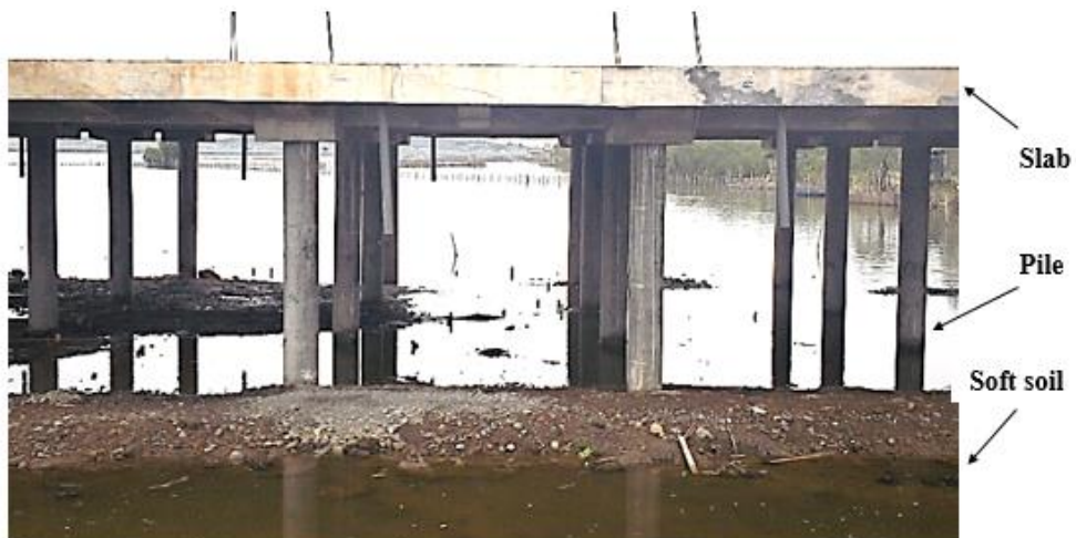
Fig. 3 - Soft soil handling with pile slab
