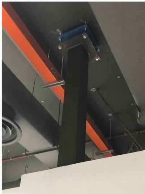
Fig. 5 - Actual LEB with 200 mm x 200 mm installed at steel columns
